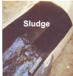
When a tank is pumped out, some oil and most of the sludge is left behind to prevent pumps from being clogged. The remaining sludge must be cleaned to ensure that the decommissioned tank is truly no longer an environmental hazard.
