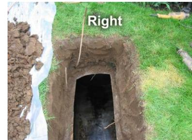
When we decommission a tank, we clean the interior of the tank and properly dispose of the oil & sludge with a DEQ approved environmental recycler. As the tank continues to rust, you do not have an environmental cleanup later. **Our decommissionings are certified with the DEQ.**
